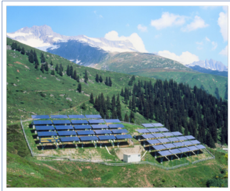
Figure 1. Solar panel array located in the Alps above Disentis, Switzerland (Bond)
